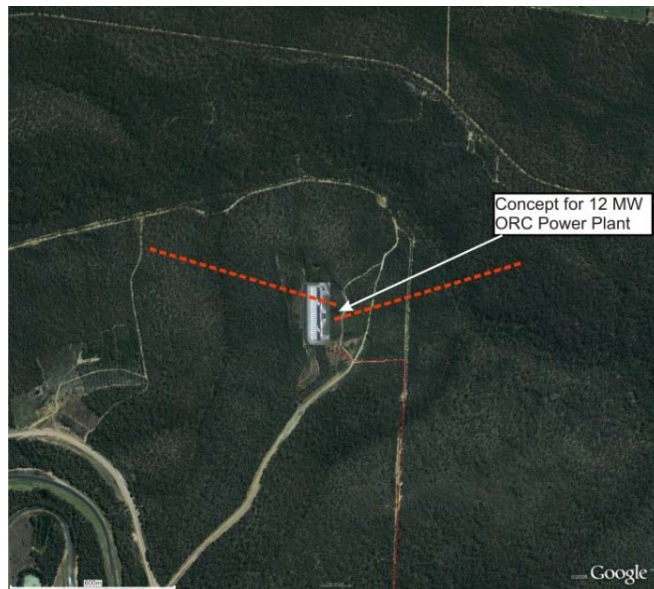
Figure 1: Aerial up view of proposed production and injection wells and ORC 12 MW e power plant
