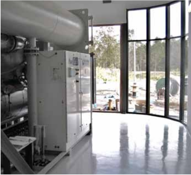
Figure 5: 280kW Purecycle ORC power system installed at Gympie Timber to convert sawmill residue into electricity
