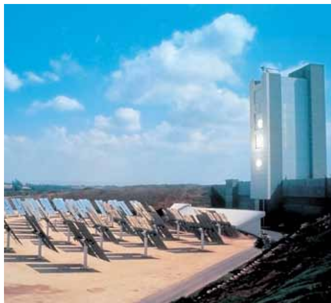
Figure 7: The Weizmann Institute of Science's Solar Tower and Field that are used in the CO 2 to Fuel Conversion Technology
