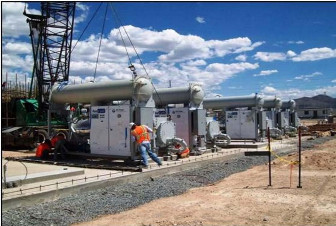
**Installation of multiple PureCycle® units**
